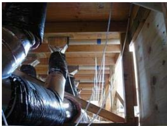
Figure 3. Ducts in the crawlspace below the test chamber.
