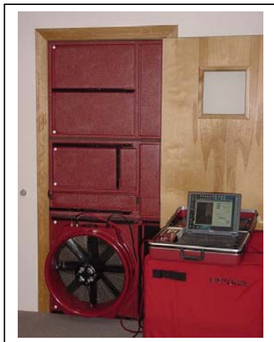
Fig.1 Door-Fan set up
