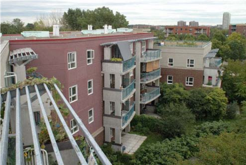
Fig 15: Balconies separately supported from the building
