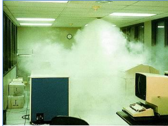
Figure 1: The Clean Agent expands causing cooling which condenses moisture to form a fog.
