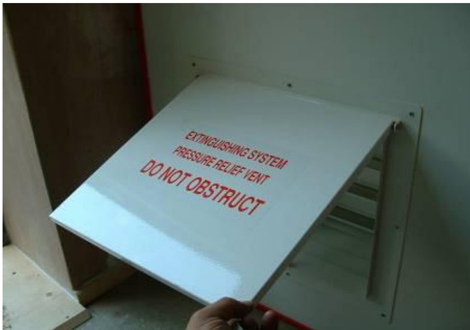
Figure 9: The sign says "DO NOT OBSTRUCT", because it is very likely the vent path will be obstructed thus the vent path must be checked regularly.
