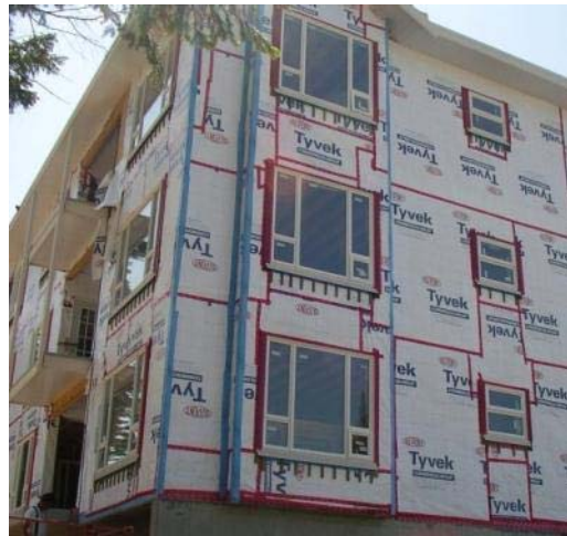
Fig.2.15 Sealed Sheathing Membrane Air Barrier Approach. When properly detailed and supported, the sealed exterior sheathing membrane air barrier approach can be a successful strategy for airflow control in a MURB. Notice the use of tapes to seal the sheathing membrane for this 4-storey wood-frame MURB. Rigidity and support of the membrane will be added in form of vertical wood strapping used to create the cavity for a rainscreen wall assembly.
