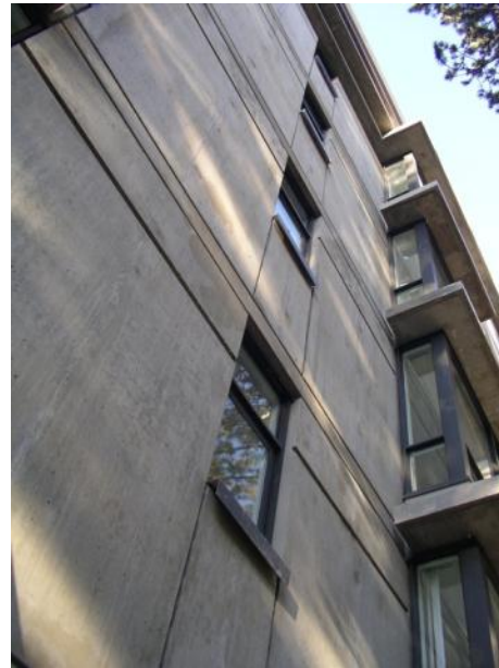
Fig.2.22 Mass Concrete Walls. Concrete and joint sealants perform the air barrier function. The proper control of cracks and joints also required for water penetration control will lead to airtight assemblies.
