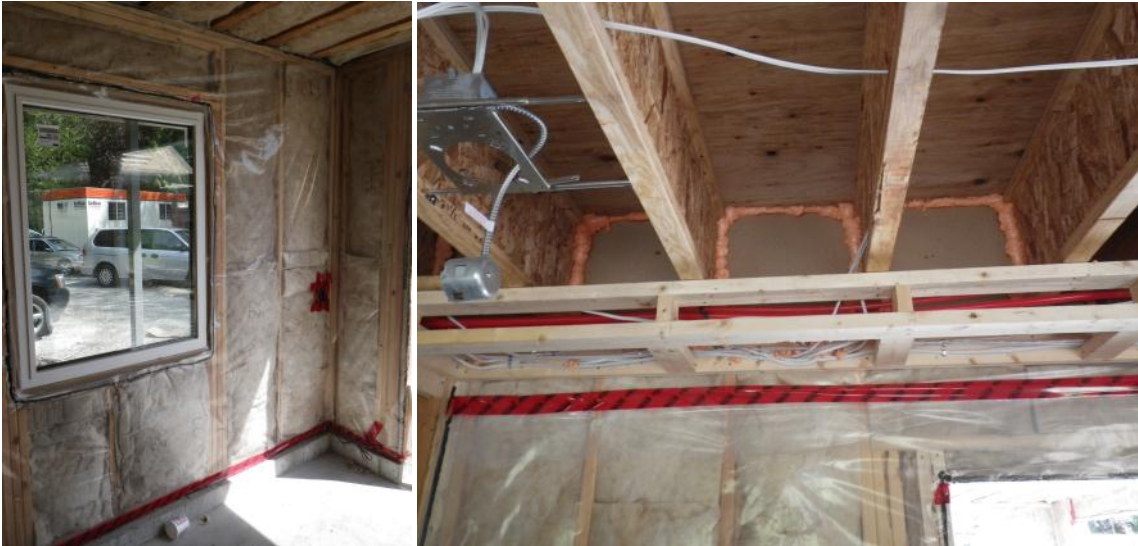
Fig.2.12 Sealed Polyethylene Approach. Utilizes acoustic sealant and construction tape for joints, details, and transitions. This approach often relies on other elements such as the rigid insulation and sprayfoam between floor joists to transition between floors. Industry familiarity with this approach and combined vapour barrier function means that many designers will elect to use this approach in designs even while not appropriate, such as when required to accommodate loadings in taller and more exposed MURBs.
