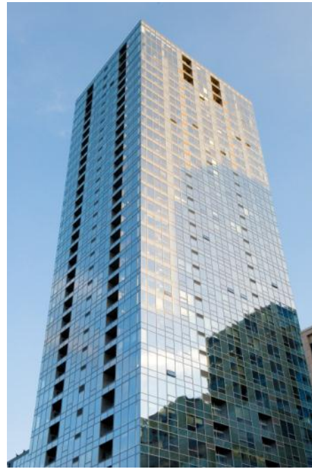
Fig.2.23 Window wall (Left) and Curtain wall (Right) assemblies occupying the majority of the vertical enclosure area of these MURBs. The air barrier system of these wall assemblies is achieved by the gaskets and sealants between the joints and interfaces of these manufactured window assemblies and interfaces to other components including slab edges.
