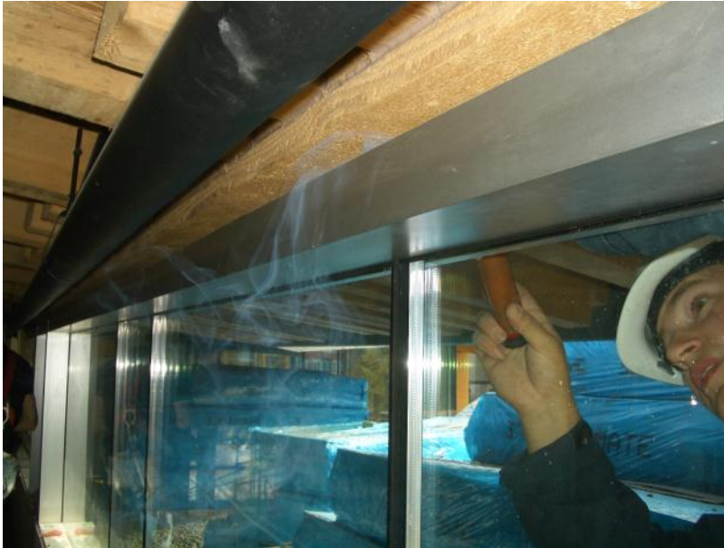
Fig.5.6 Smoke Wand to Detect Leak and Direction of Airflow at Interface Detail
