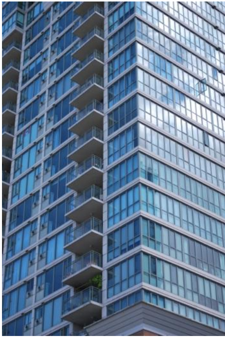
Fig.2.23 Window wall (Left) and Curtain wall (Right) assemblies occupying the majority of the vertical enclosure area of these MURBs. The air barrier system of these wall assemblies is achieved by the gaskets and sealants between the joints and interfaces of these manufactured window assemblies and interfaces to other components including slab edges.
