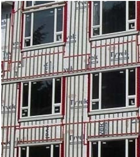
Fig.2.17 Supported Sheathing Membrane Approach with Vertical Strapping/Girts. Exterior sheet air barrier membrane with vertical wood strapping or metal girts more evenly distributed loads and deflection of the membrane. There is very little test data available to allow for a more analytical or even empirical approach to the determination of structural adequacy for sheet membrane barrier systems. Precautionary measures could include tightly spaced strapping to secure the membrane and selection of more robust membrane, with respect to both strength and tear-resistance. The use of self-adhered and liquid membranes basically makes the sheathing and membrane an integral, rigid air barrier material.
