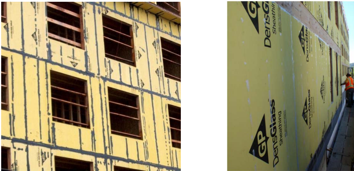
Fig.2.14 Sealed Sheathing Approach. This approach utilizes the rigid exterior sheathing sealed with sealants, membranes or tapes. The system provides good performance for all MURB heights due to rigidity, ease of inspection and detailing.
