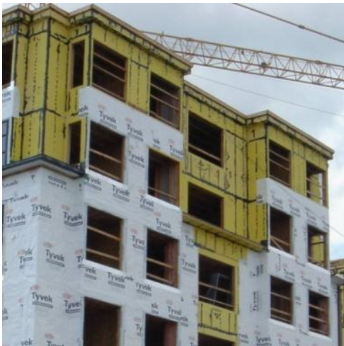
Fig.2.13 An exterior air barrier approach can be utilized to either seal the joints in the exterior sheathing or seal the exterior sheathing membrane. Selection of which component to seal will depend on cladding type, MURB height and contractor familiarity with the approach.
