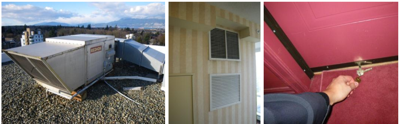
Fig.2.9 Rooftop Make-up Air Unit, Corridor Supply Grille, and Door Undercuts Utilized as Part of the Pressurized Corridor Air Distribution System in Most MURBs
