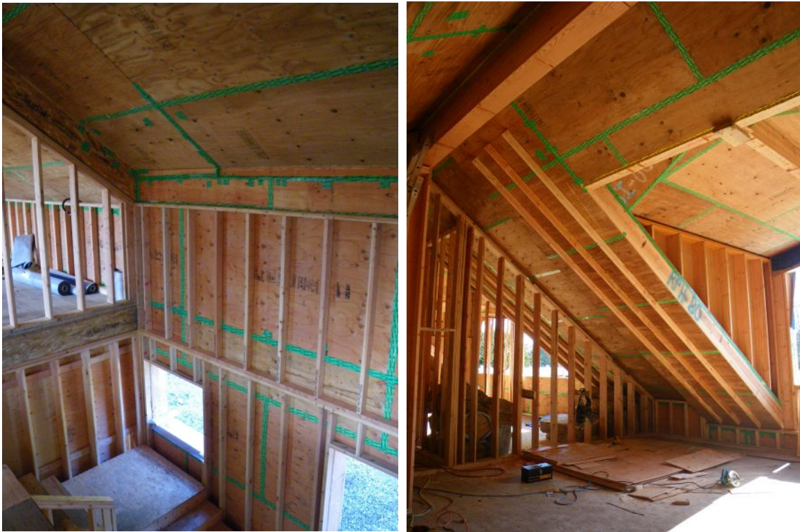
Fig.2.24 Taped Plywood Sheathing as the Interior Air barrier System of Pre-fabricated Wood-panels. Durable and long-lasting tapes must be used to maintain airtightness over the life of the building.
