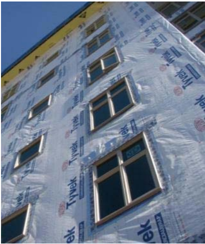
Fig.2.15 Sealed Sheathing Membrane Air Barrier Approach. When properly detailed and supported, the sealed exterior sheathing membrane air barrier approach can be a successful strategy for airflow control in a MURB. Notice the use of tapes to seal the sheathing membrane for this 4-storey wood-frame MURB. Rigidity and support of the membrane will be added in form of vertical wood strapping used to create the cavity for a rainscreen wall assembly.
