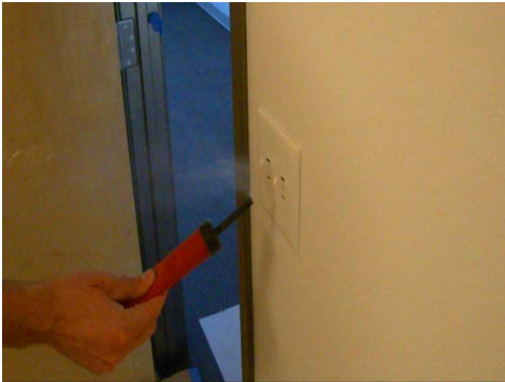
Fig.5.11 Smoke Wand Being Used to Show Airflow Out of Electrical Outlet
