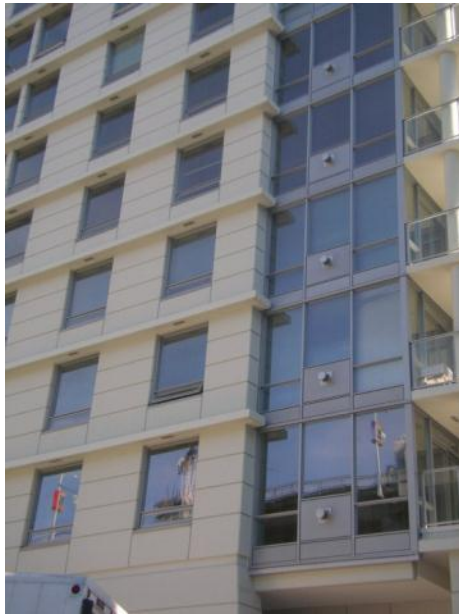
Fig.2.22 Mass Concrete Walls. Concrete and joint sealants perform the air barrier function. The proper control of cracks and joints also required for water penetration control will lead to airtight assemblies.
