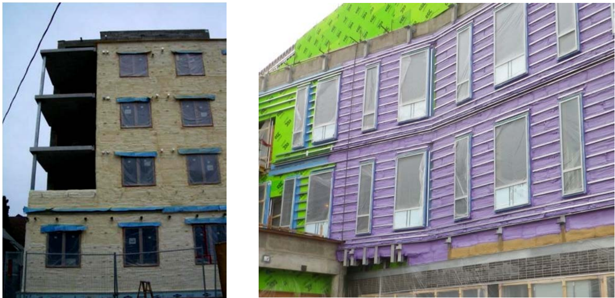
Fig.2.20 Closed Cell Sprayfoam Applied on the Exterior of the Exterior Sheathing/Back-up Wall as the air barrier strategy for these walls. Appropriate self-adhered membranes are used to transition between the foam and penetrations including windows.
