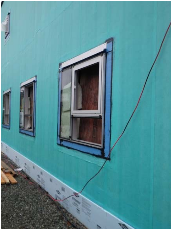
Fig.2.18 Self-Adhered Vapour Permeable Air Barrier Membrane on Plywood. The membrane performs the function of the WRB/sheathing membrane and when adhered to the plywood provides a rigid air barrier system suitable for taller wood-frame MURBs regardless of cladding strategy.
