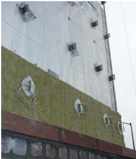
Fig.2.16 Sealed Sheathing Membrane Air Barrier Approach with Brick Ties. A limitation of the sealed sheathing membrane approach is the potential for the air barrier membrane (and WRB) to tear or become damaged around brick-tie penetrations. Solutions include SAM reinforcement over the sheathing membrane at the fastener locations or use of self-adhered and liquid membranes.
