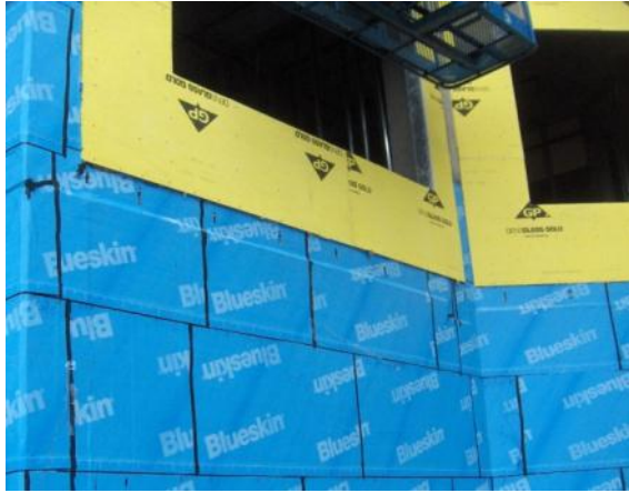
Fig.2.19 Self-Adhered Membrane (SAM) Air Barrier Membrane Applied to Fiberglass Faced Gypsum Sheathing. The simplicity of this system and use of exterior insulation makes this air barrier system common for non-combustible high-rise MURB construction and in particularly for exterior enclosure rehabilitations.
