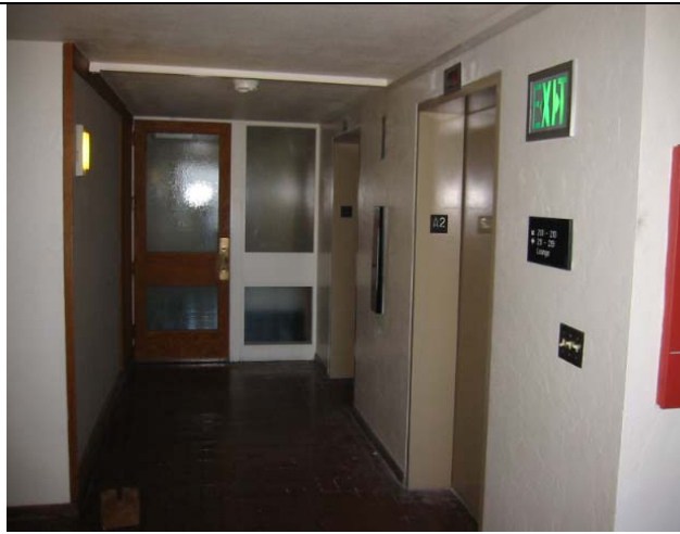
Vestibule in hallway isolates enclosed stairwell and elevator doors.
