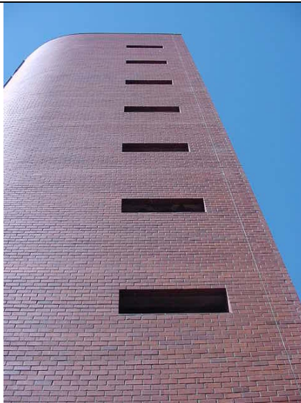
Windowless vent holes in stairwell used for testing.
