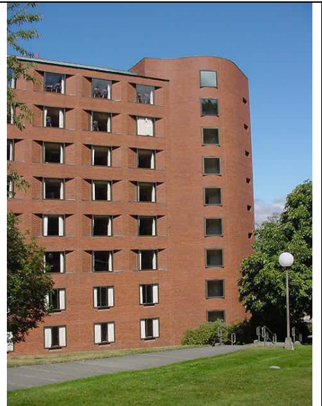
Back of building show the 8 floors that were tested in units of two floors at a time.
