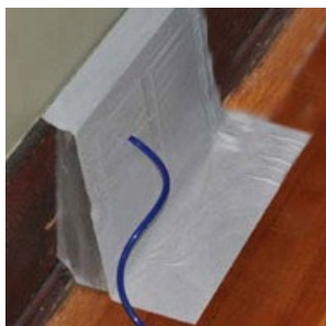
Figure 10: Seal all supply and return registers with Grill Mask
