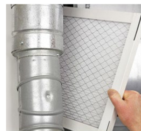
Figure 11: Remove all air filters
