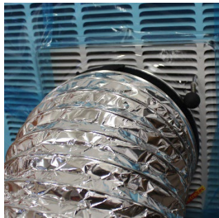
Figure 18: Flex Duct connected to the Flange.
