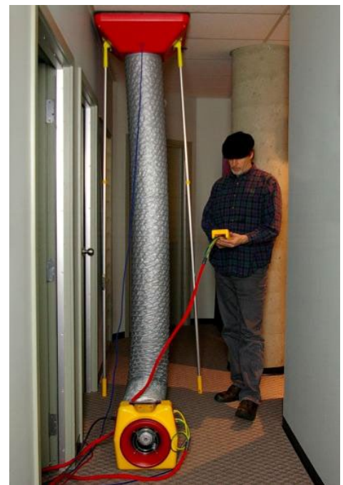
Figure 38: Measuring air flow with a Powered Flow Hood
