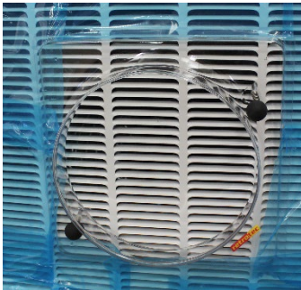
Figure 19: Flange taped onto a return register before attaching the Flex Duct
