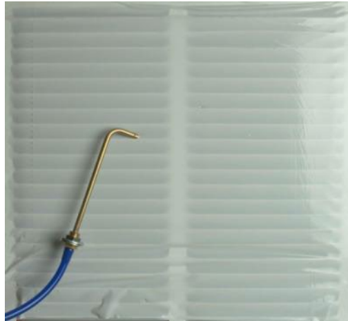
Figure 16: Insert the blue tube into a supply register closest to the air handler
