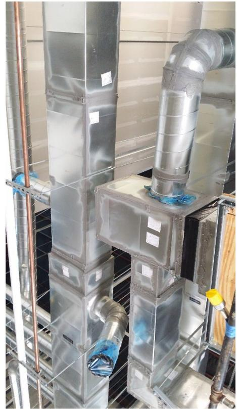
Select a limited section of duct that you have sufficient power to test. Measure the duct surface area in square feet.
