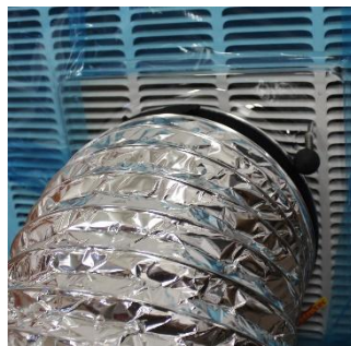
Figure 18: Flex Duct connected to the Flange.
