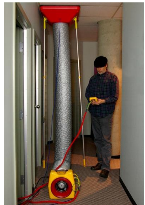
Figure 26: Measuring air flow with a Powered Flow Hood
