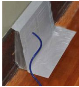
Figure 9: Seal all supply and return registers with Grill Mask
