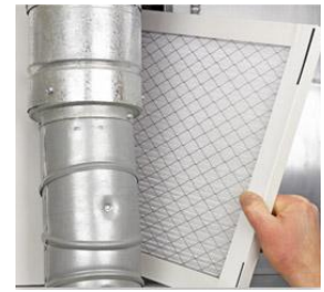
Figure 10: Remove all air filters
