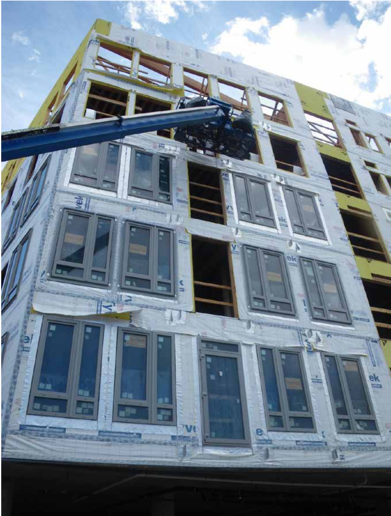
Wood-frame building over concrete podium, designed to allow completion of the air barrier before balconies are installed on clips
