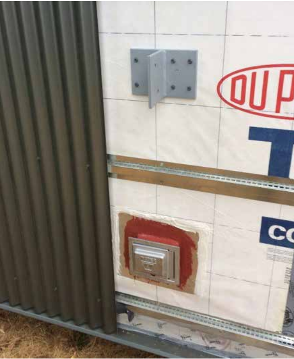
Mock-ups of various wall penetrations
