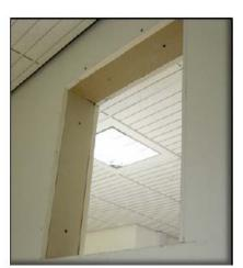
e) Mark the flange through which the fixing screws will seat into the framing studs.
