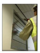
g) Mark and drill the wall liner flange as per PRV flange. Apply a bead of intumescent fire-rated caulk around the opening face where the wall liner flange is to fit or around the wall liner flange and fix in with 3 inch (75mm) no. 6 steel screws.
