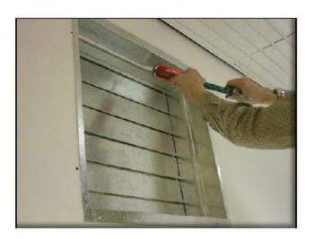
i) Check that each and every blade of the PRV opens freely. If blades are rubbing against the side casing check to make sure the frame of the PRV has been fitted square and is not twisted and there is no part of the wall opening that is jamming on the vent casing. (it may be possible to free slightly rubbing blades by tapping out casing where they touch, with a hammer).
