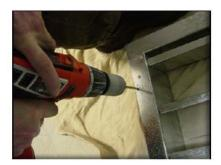
f) After checking to make sure the PRV and the Wall Liner fit, run a bead of intumescent fire-rated caulk around the face of the wall opening so as to form a seal under the PRV flange and using 3 inch (75mm) long no. 6 steel screws fix the PRV into the hole.
