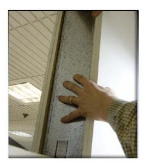
d) The opening must be framed out with similar studs that the wall is made from, e.g. if cutting into a 2hour fire rated wall with steel studs then steel studs must be used to frame the hole so as to maintain the 2 hour fire rating. The frame must then be lined with Plasterboard.
