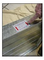
b) Measure the PRV wall liner and add a 1/2 inch (12mm) to the measurement mark out and cut a hole into the stud partition. (Note that the larger of the measurements is always the width).
