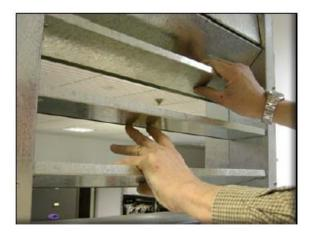
j) Hold grill over PRV flange and fix using 1 inch (25mm) tech screws. Do not over tighten screw since they can distort grill frame. Do the same for Wall liner.
